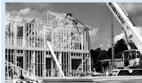
Trusses set on August 1
